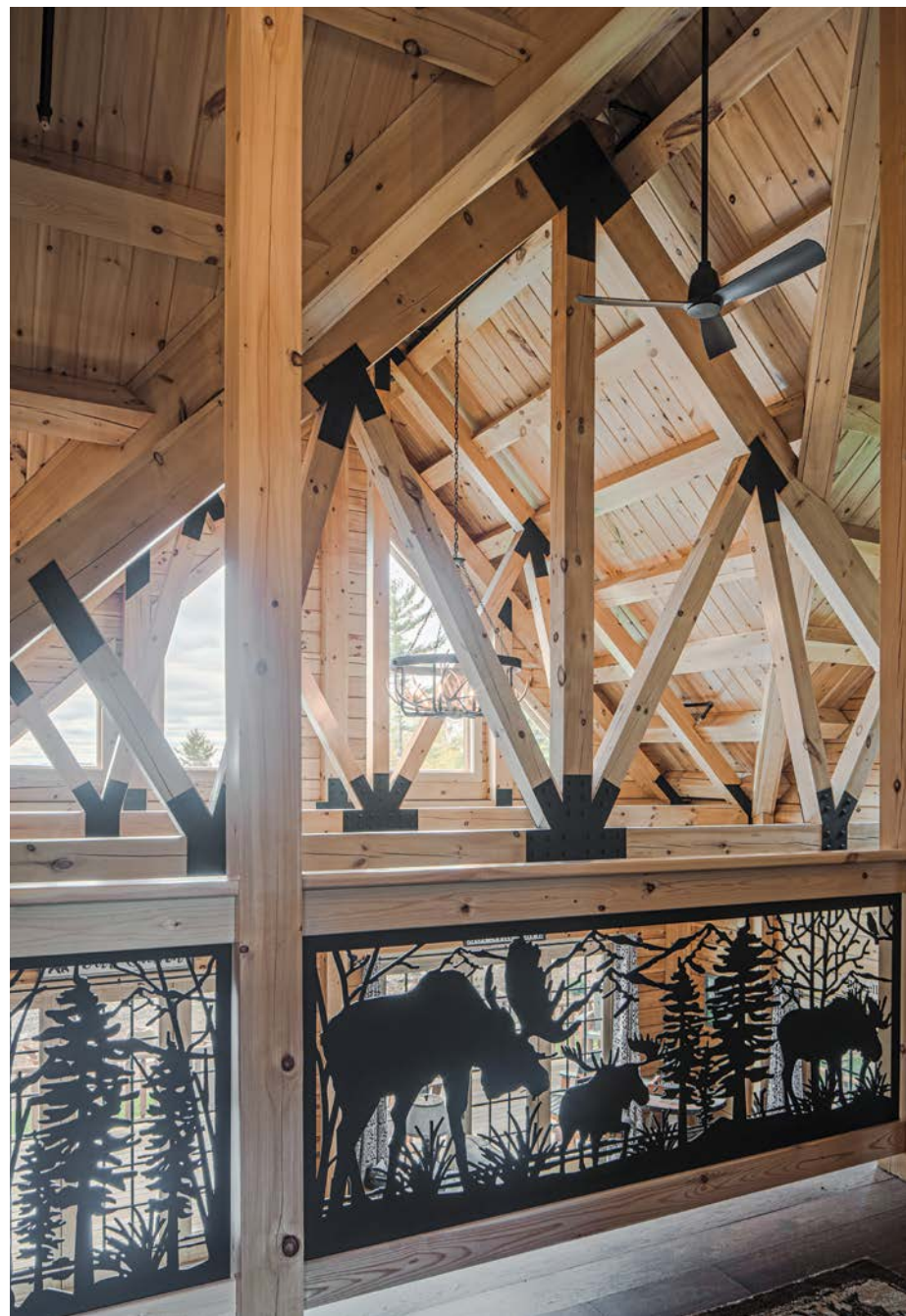
above Black, laser-cut steel accents on the loft railing pop against the clear-acrylic-stained eastern white pine timbers and tongue-and-groove in Coventry's Craftsman-style purlin-and-truss roof system.
